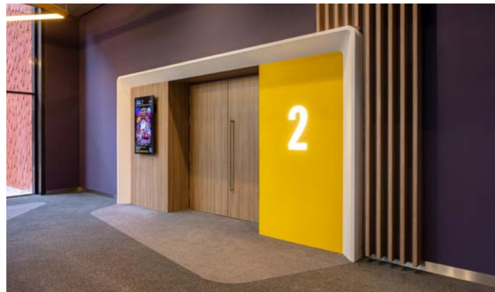
The large, flush-mounted hall numbers are illuminated from behind to aid orientation in a discreet way.
